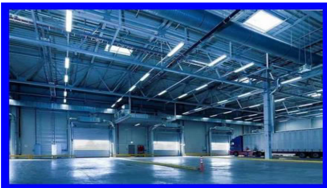
Industrial Lighting ( Bajaj )
